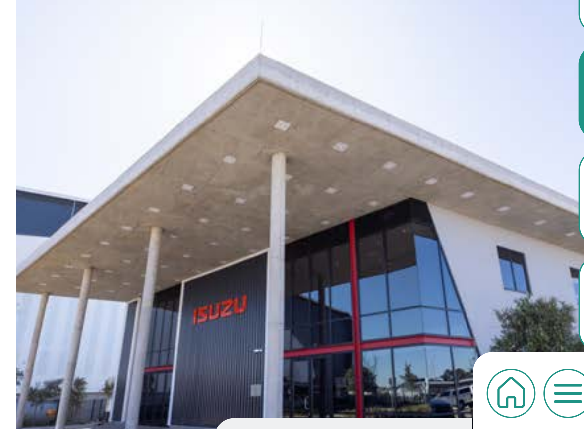
S&J Industrial Park, Gauteng, South Africa
